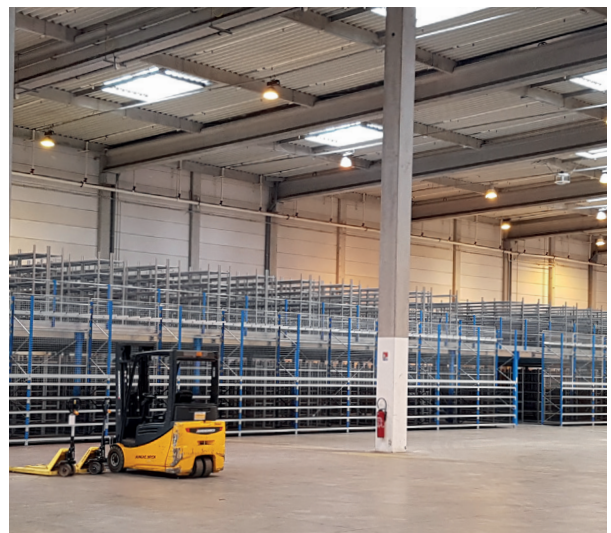
Large-scale installation combining shelving and mezzanine floor.
